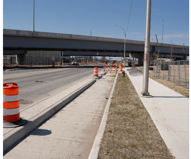
Fort Street local road improvement progress.
