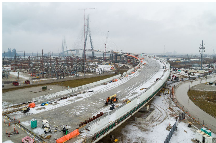
Construction progress of the Gordie Howe International Bridge.
