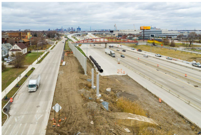
Construction progress of the I-75 work.
